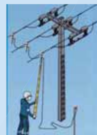
Lifting earthing devices
